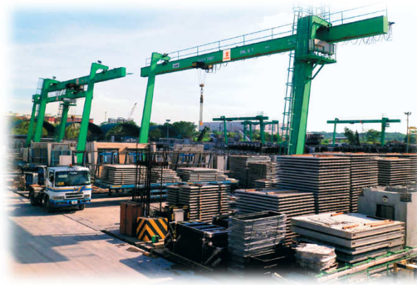
Precast Yard in Singapore
